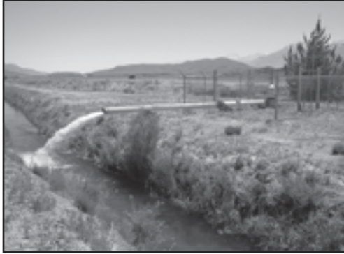
Pumping groundwater in Big Pine
